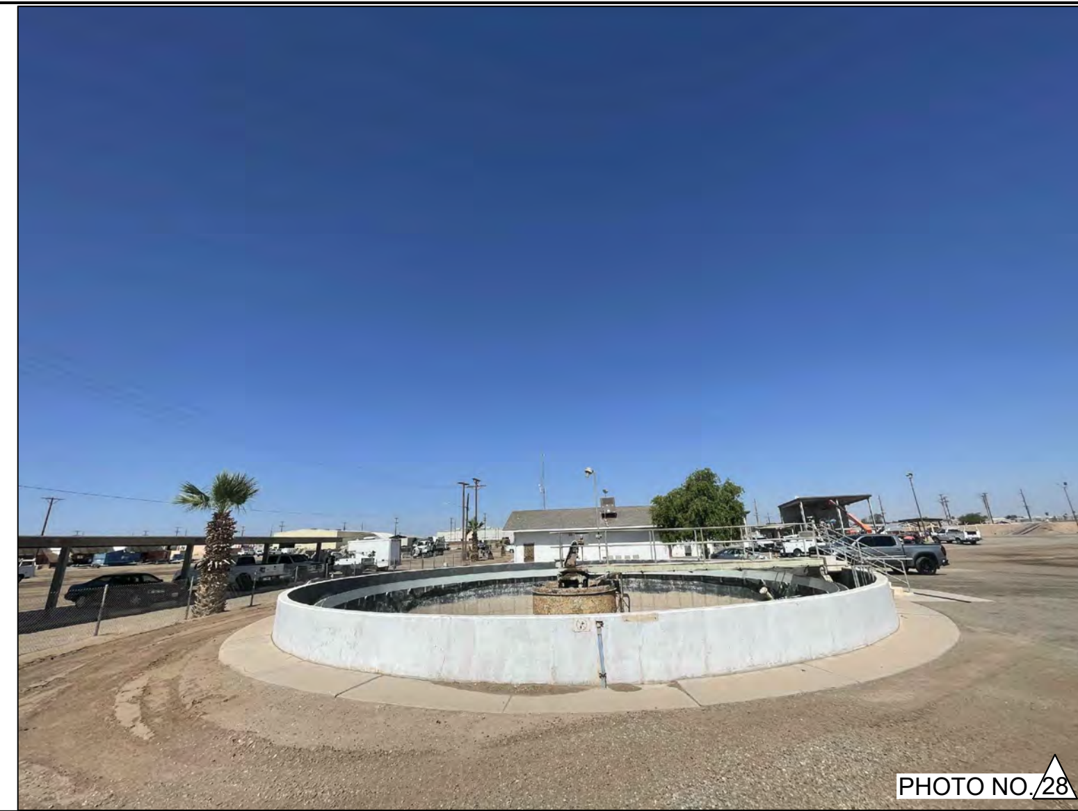
CLARIFIER NO. 1 - PHOTO OF THE EAST SIDE VIEW OF CLARIFIER NUMBER 1.
