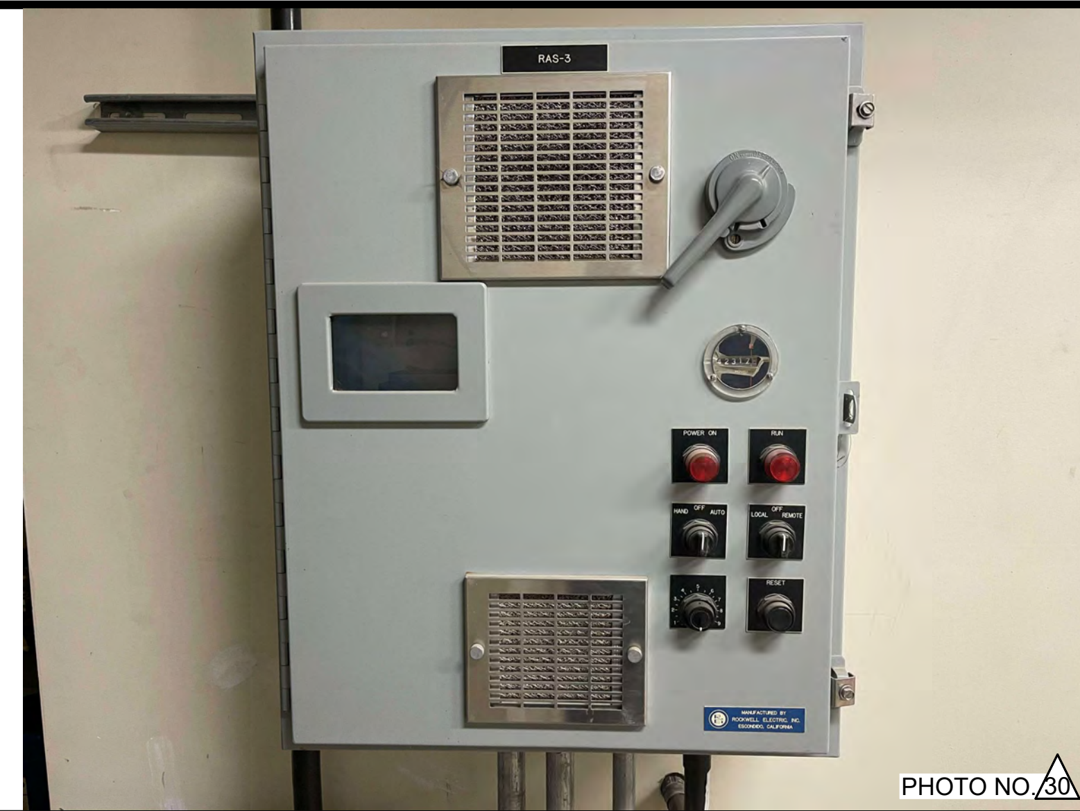
PHOTO OF RAS-3 ELECTRICAL PANEL AT THE NORTH WALL OF SLUDGE PUMP STATION UPPER FLOOR.
