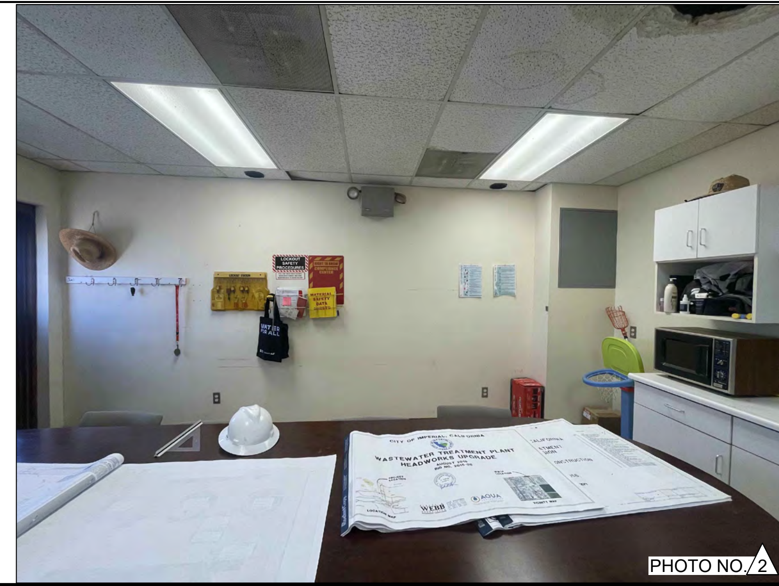
OPERATIONS BUILDING - PHOTO OF THE EAST WALL OF EXISTING BREAK ROOM.
