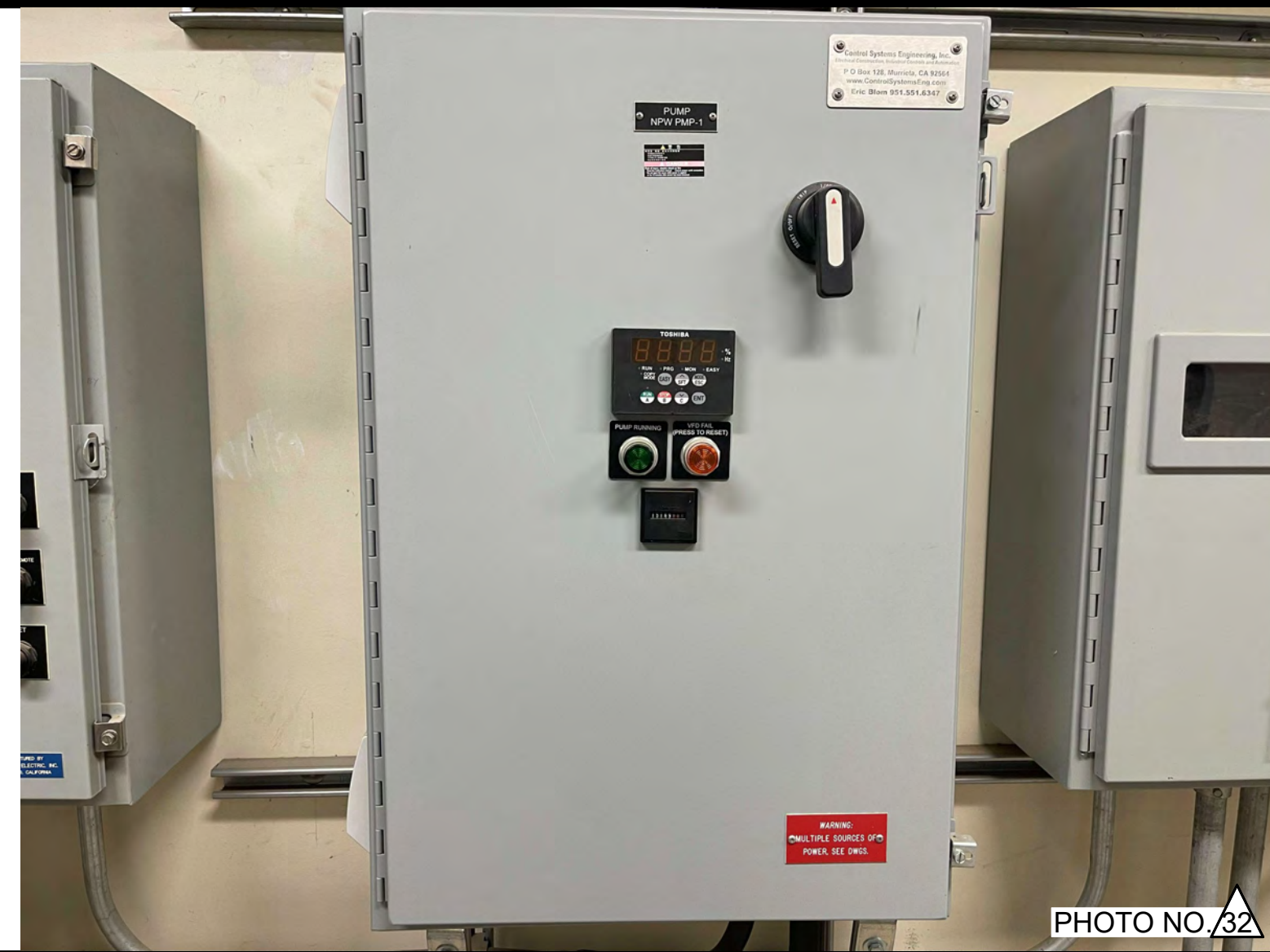
PHOTO OF NON POTABLE WATER PMP-1 ELECTRICAL PANEL AT THE NORTH WALL OF SLUDGE PUMP STATION UPPER FLOOR.
