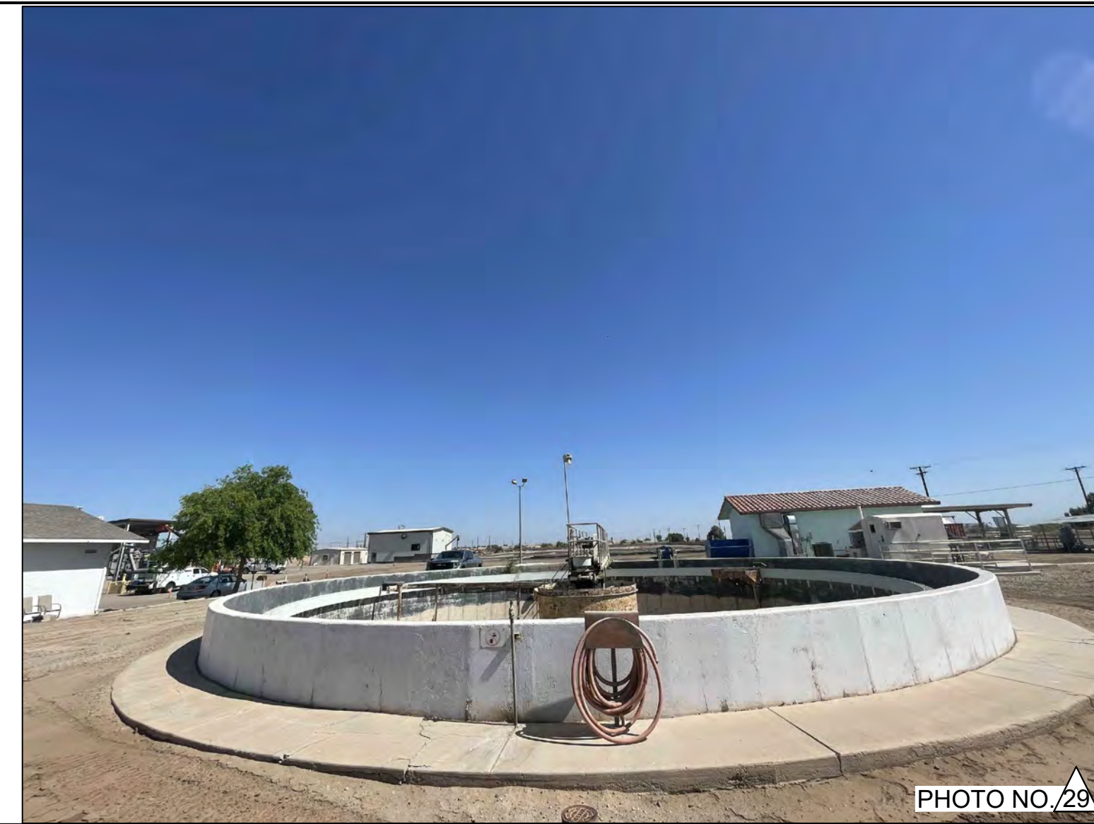
CLARIFIER NO. 1 - PHOTO OF THE SOUTH SIDE VIEW OF CLARIFIER NUMBER 1.
