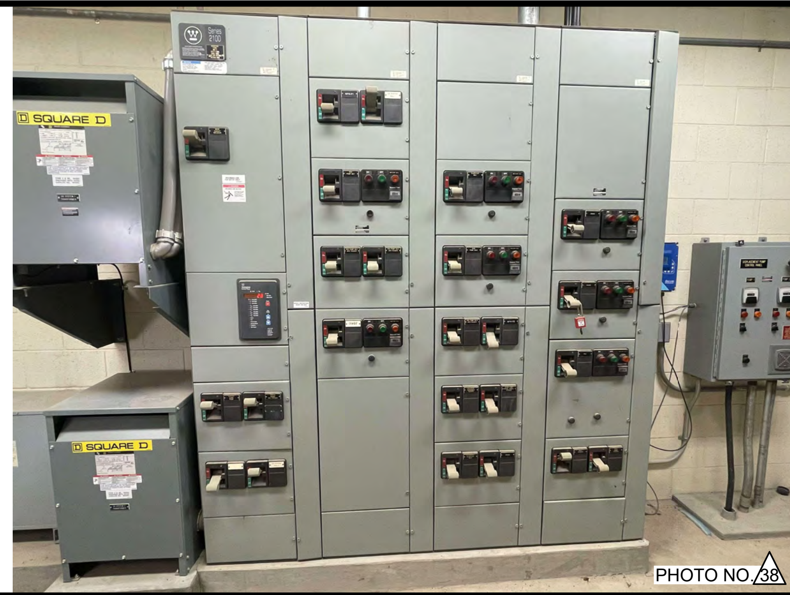
PHOTO OF THE MCC WITH ON/OFF HANDLES AND INDICATOR LIGHTS, LOCATED ON THE SOUTH WALL OF THE SLUDGE PUMP STATION UPPER FLOOR.
