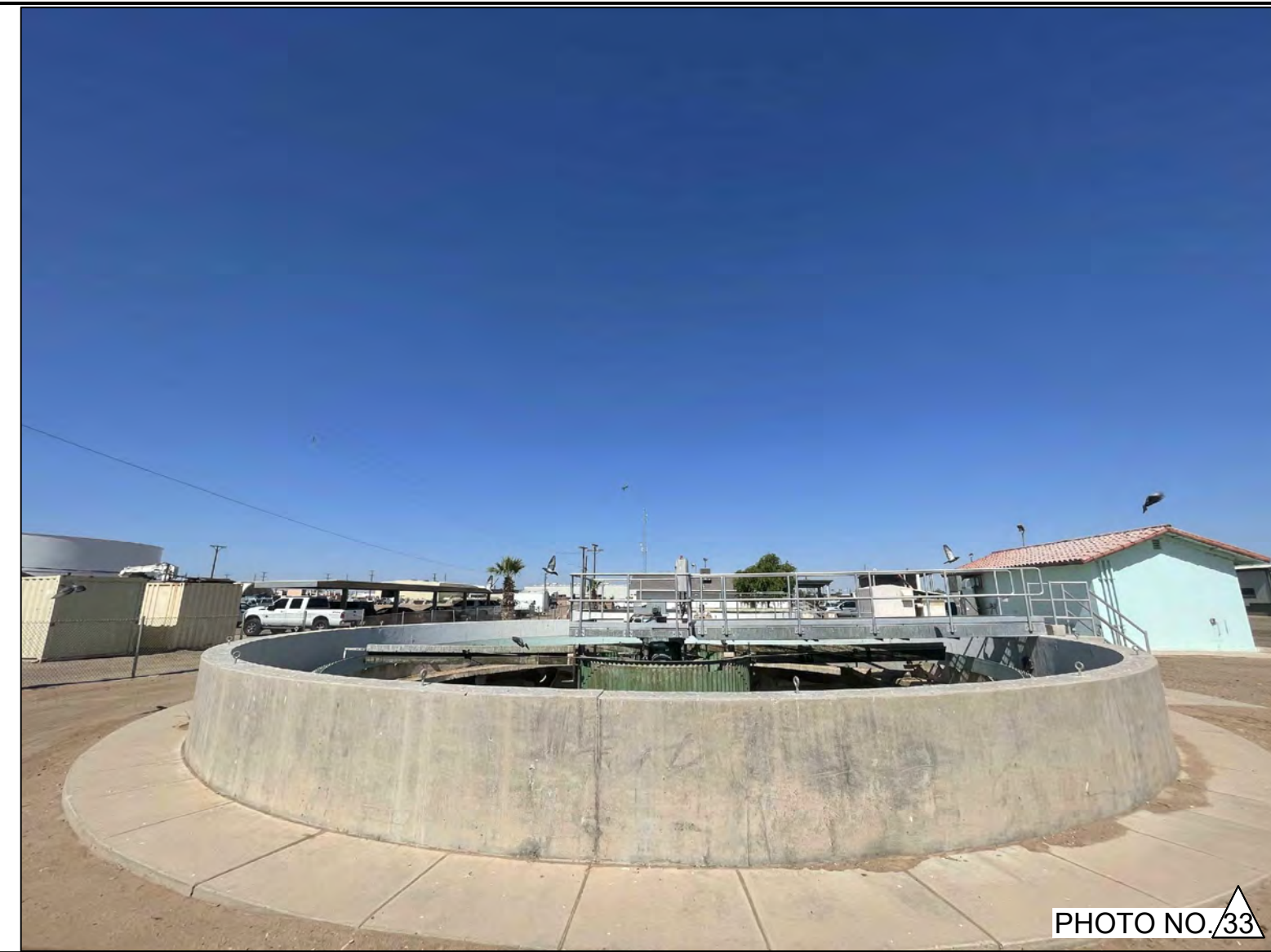
CLARIFIER NO. 2 - PHOTO OF THE EAST SIDE VIEW OF CLARIFIER NUMBER 2.
