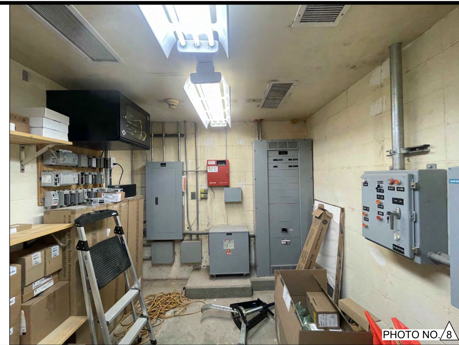
OPERATIONS BUILDING - PHOTO OF THE WEST WALL OF EXISTING ELECTRICAL ROOM.
