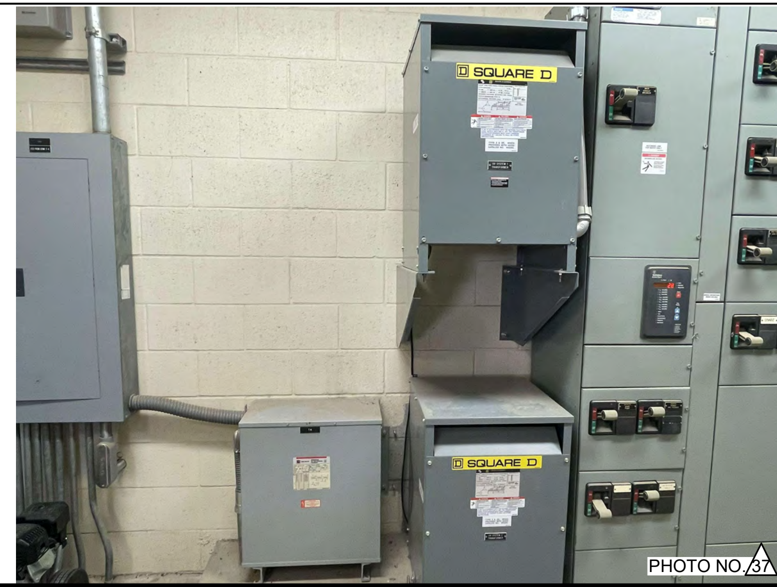
PHOTO OF BUILDING TRANSFORMER & TWO STACKED TRANSFORMERS AT THE SOUTH WALL OF SLUDGE PUMP STATION UPPER FLOOR.
