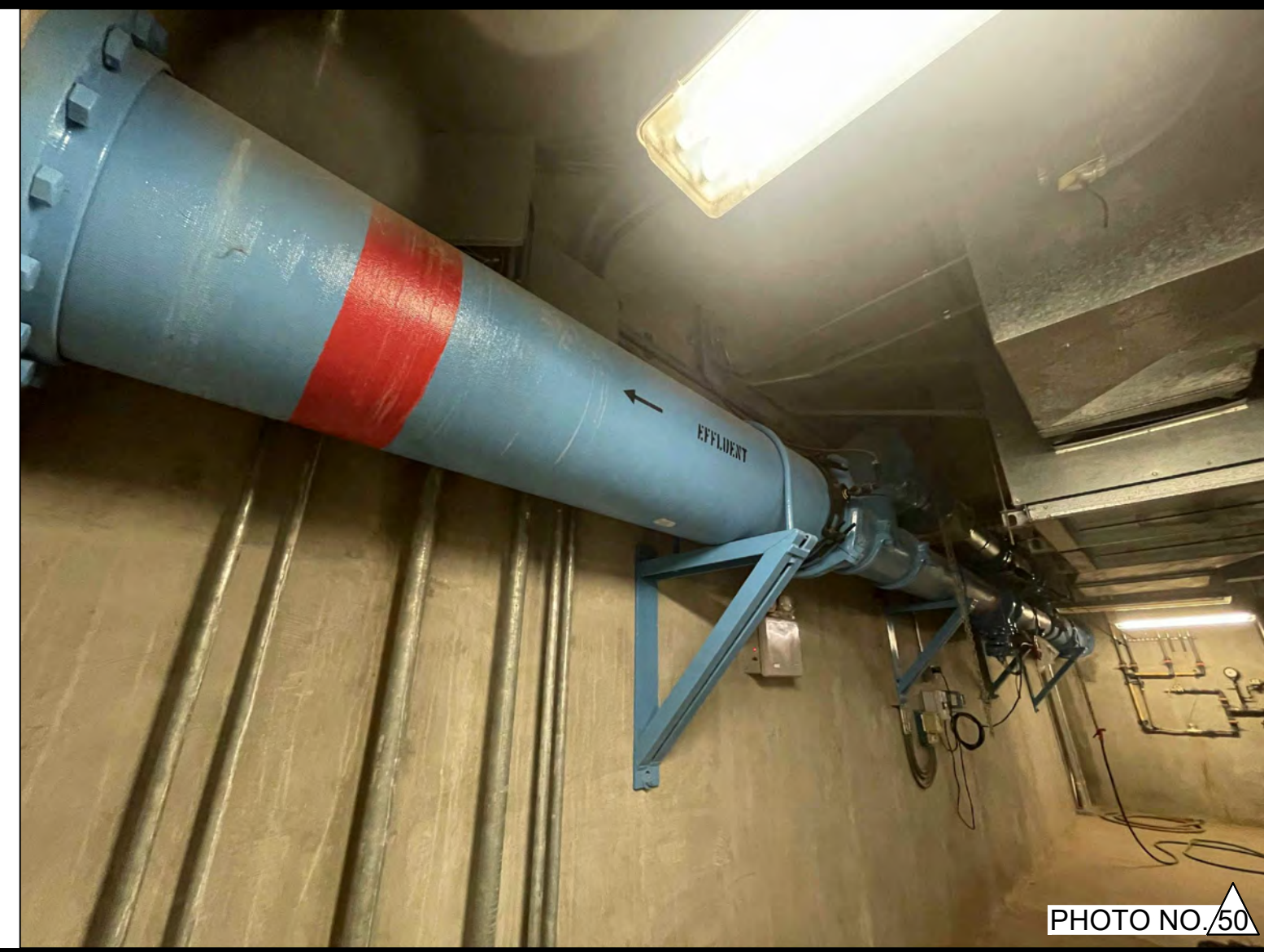
PHOTO OF THE 18-INCH AND 12-INCH PIPELINES ON THE EAST WALL OF EXISTING SLUDGE PUMP STATION LOWER FLOOR.
