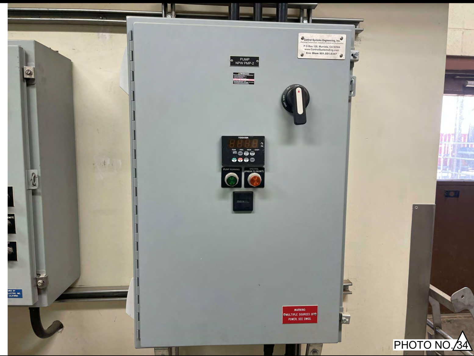
PHOTO OF NON POTABLE WATER PMP-2 ELECTRICAL PANEL AT THE NORTH WALL OF SLUDGE PUMP STATION UPPER FLOOR.
