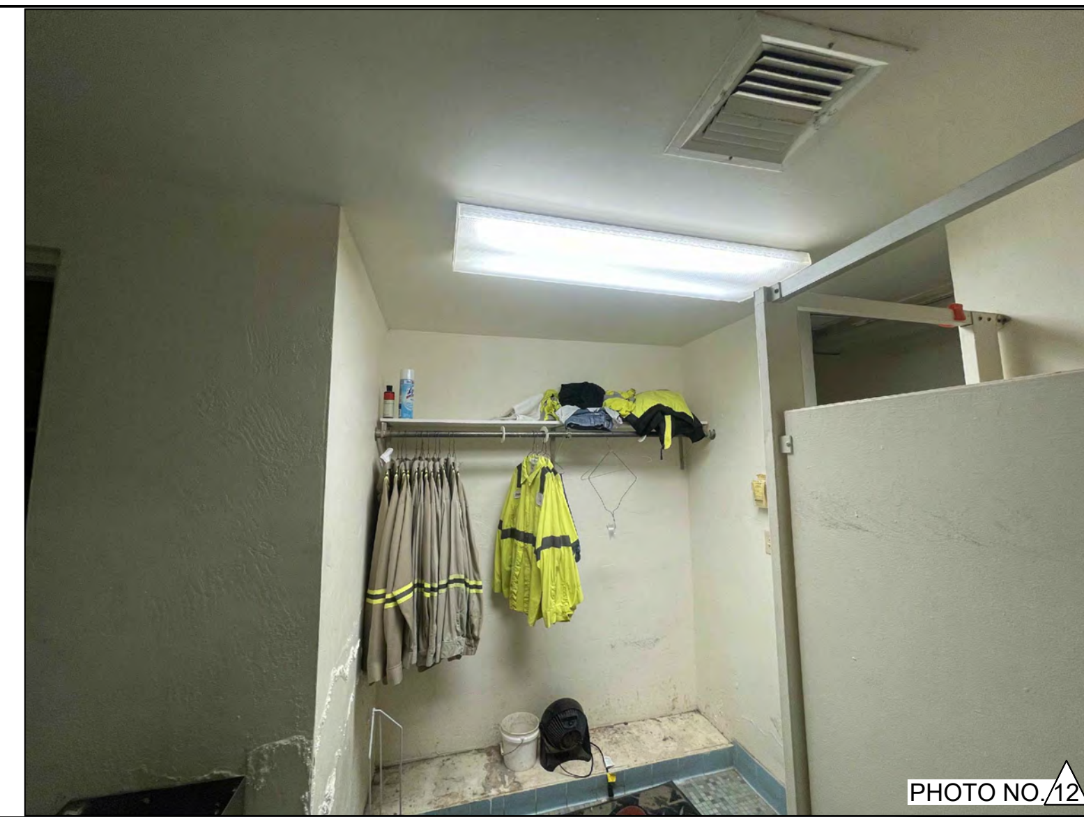
OPERATIONS BUILDING - PHOTO OF THE WEST WALL OF EXISTING BATHROOM.
