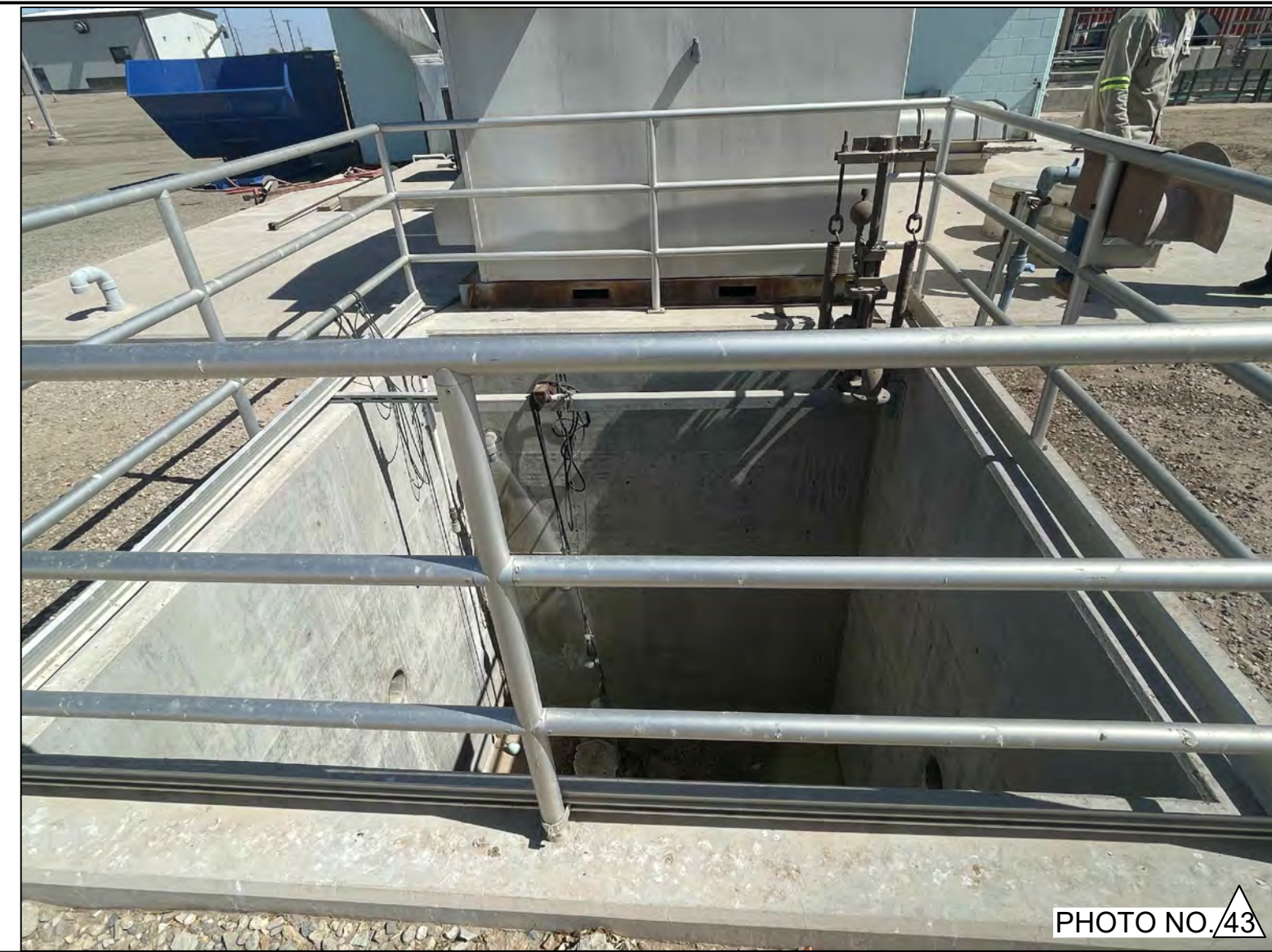
PHOTO OF THE SCUM PIT OF EXISTING SLUDGE PUMP STATION LOWER FLOOR.
