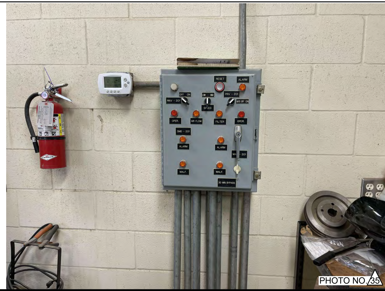
PHOTO OF BUILDING TEMPERATURE CONTROL PANEL AT THE EAST WALL OF SLUDGE PUMP STATION UPPER FLOOR.
