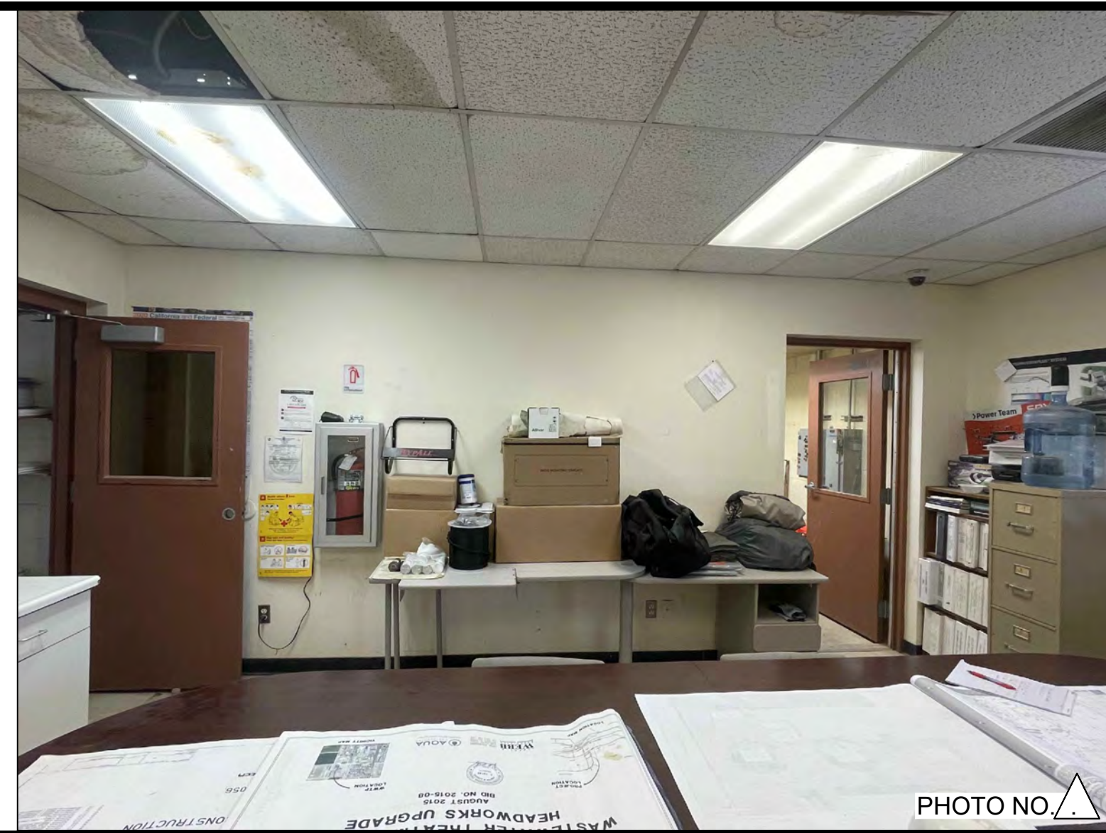
OPERATIONS BUILDING - PHOTO OF THE WEST WALL OF EXISTING BREAK ROOM.
