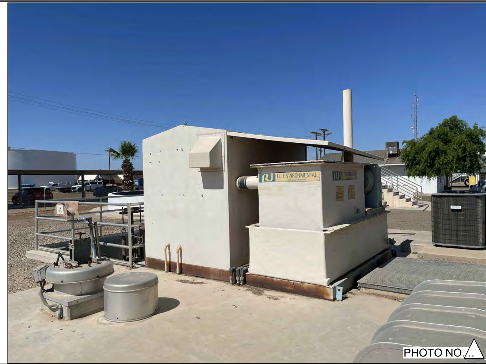
PHOTO OF THE MODULAR SCRUBBER AND CHLORINE FACILITY OF EXISTING SLUDGE PUMP STATION LOWER FLOOR.
