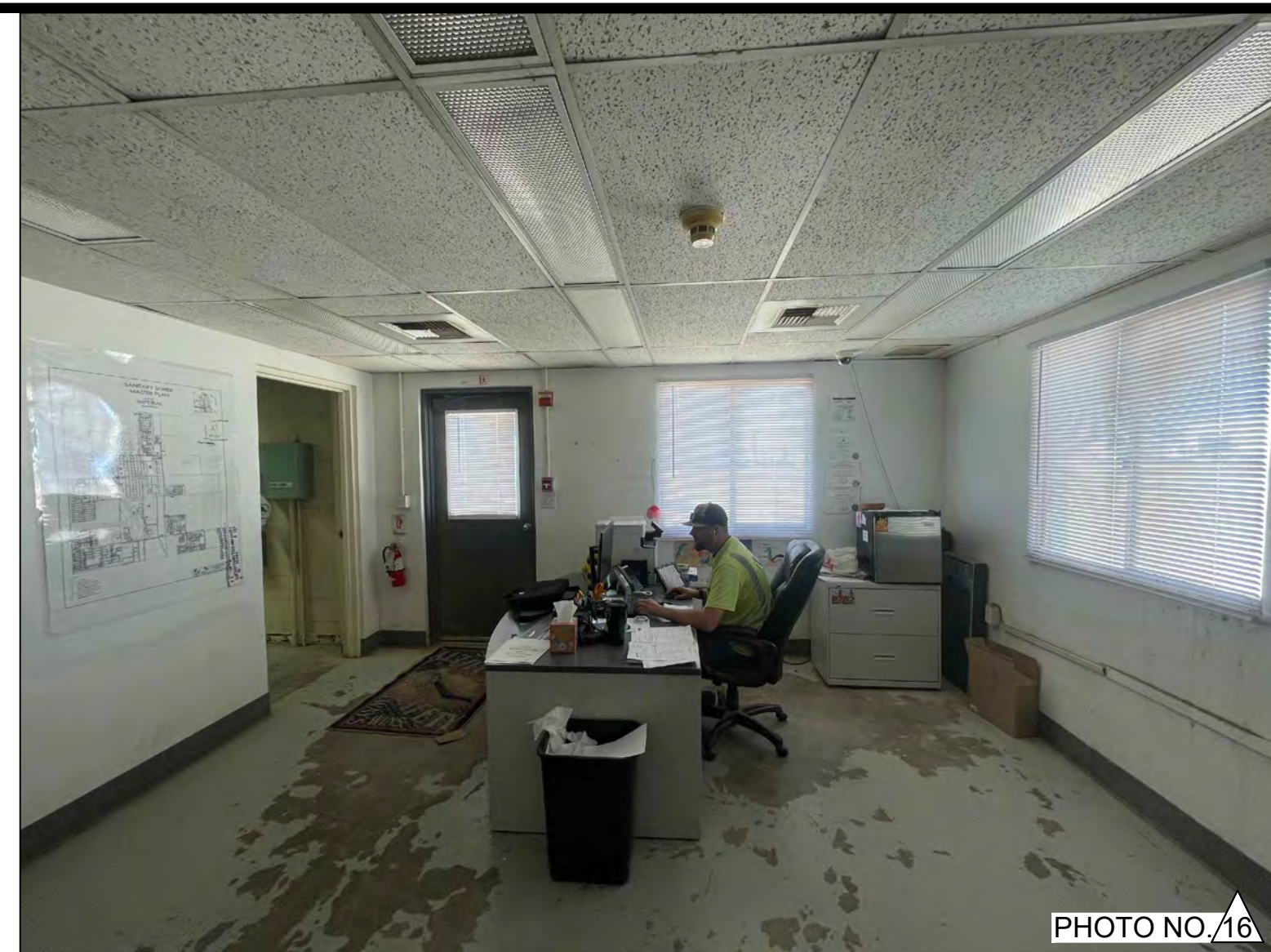
OPERATIONS BUILDING - PHOTO OF THE SOUTH WALL OF EXISTING OFFICE.
