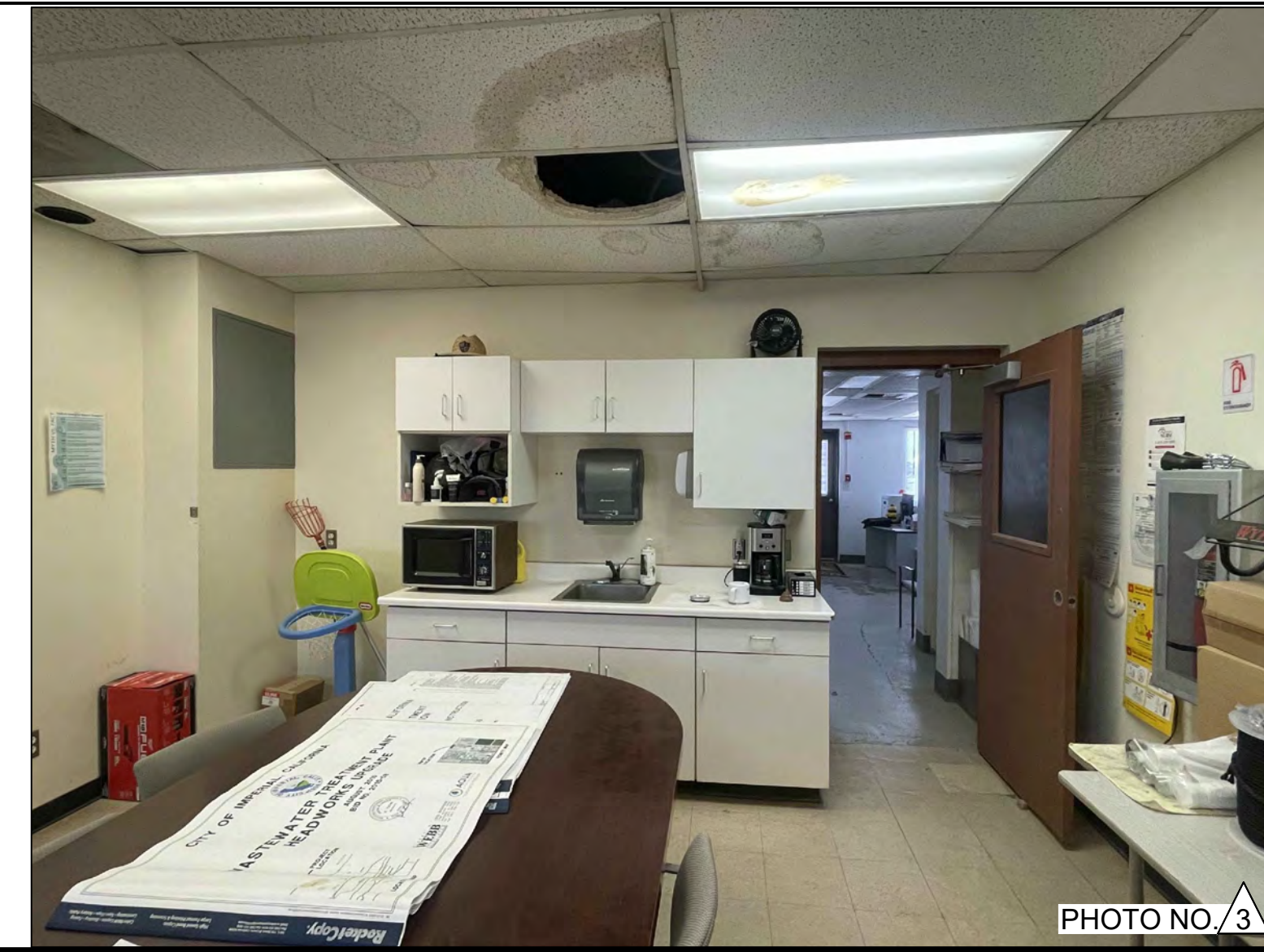
OPERATIONS BUILDING - PHOTO OF THE SOUTH WALL OF EXISTING BREAK ROOM.
