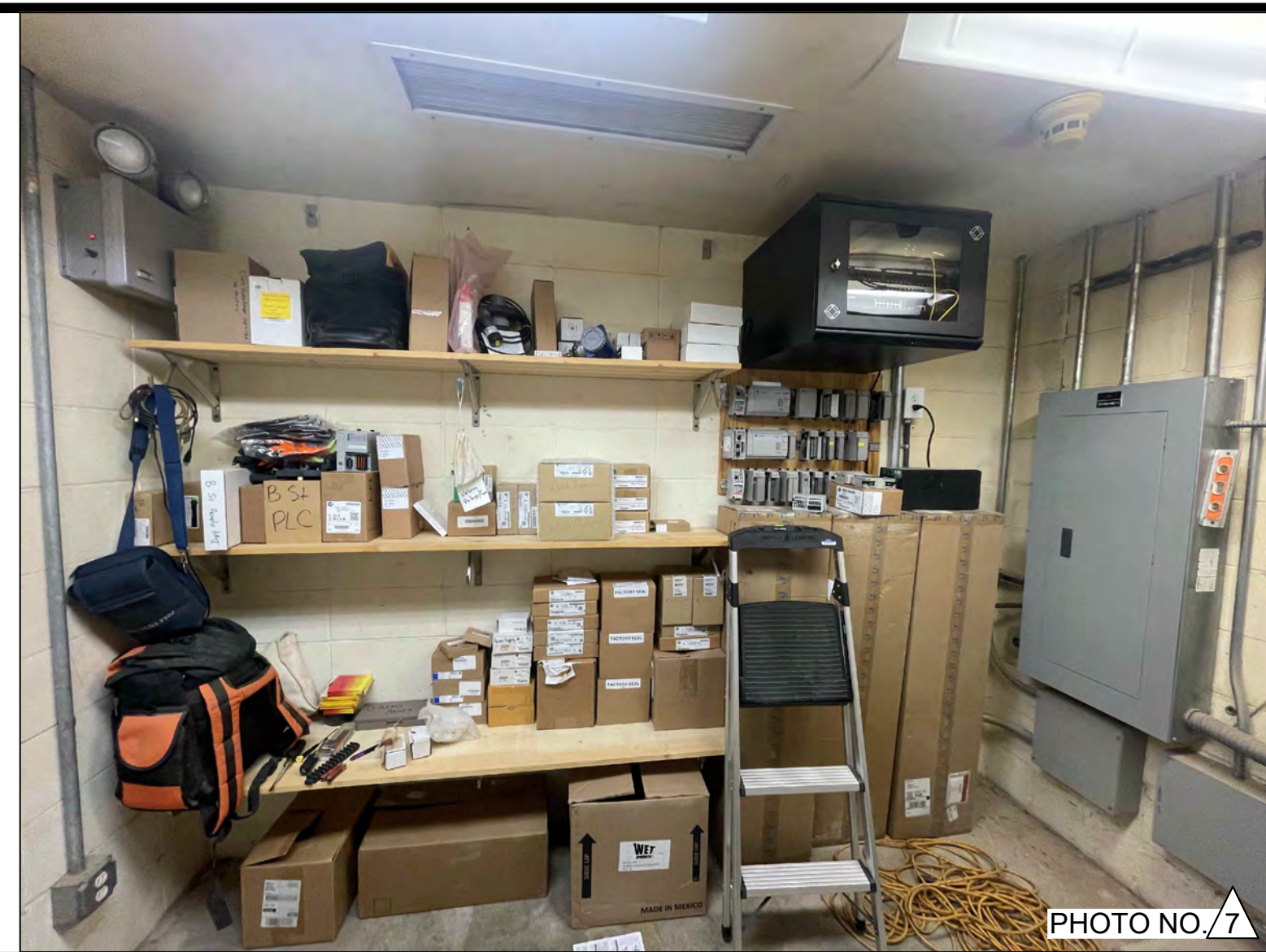
OPERATIONS BUILDING - PHOTO OF THE SOUTH WALL OF EXISTING ELECTRICAL ROOM.
