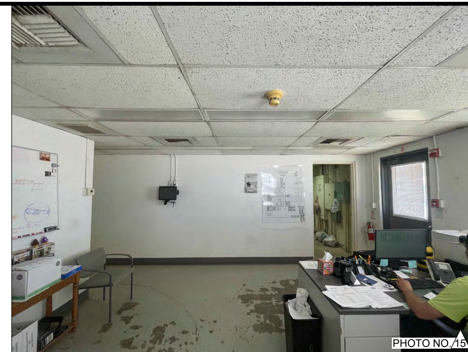
OPERATIONS BUILDING - PHOTO OF THE EAST WALL OF EXISTING OFFICE.
