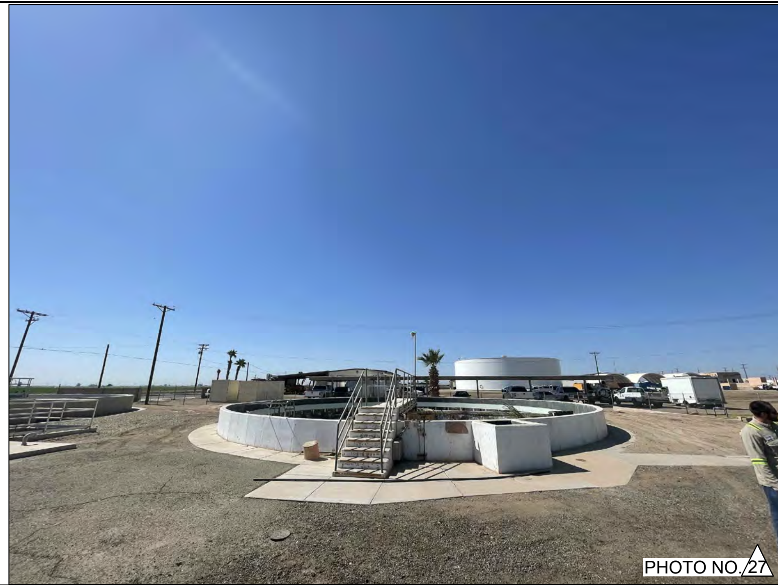
CLARIFIER NO. 1 - PHOTO OF THE NORTH SIDE VIEW OF CLARIFIER NUMBER 1.
