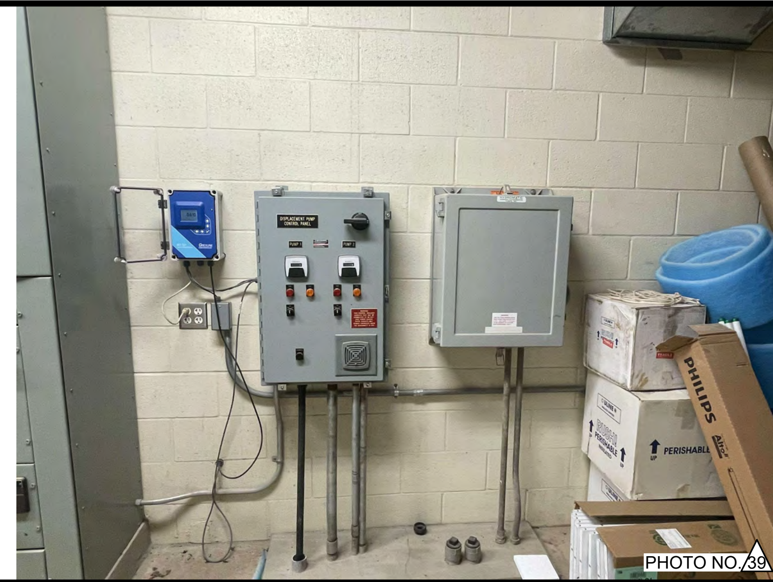
PHOTO OF DISPLACEMENT PUMP & SUMP PUMP CONTROL PANELS AT THE SOUTH WALL OF SLUDGE PUMP STATION UPPER FLOOR.
