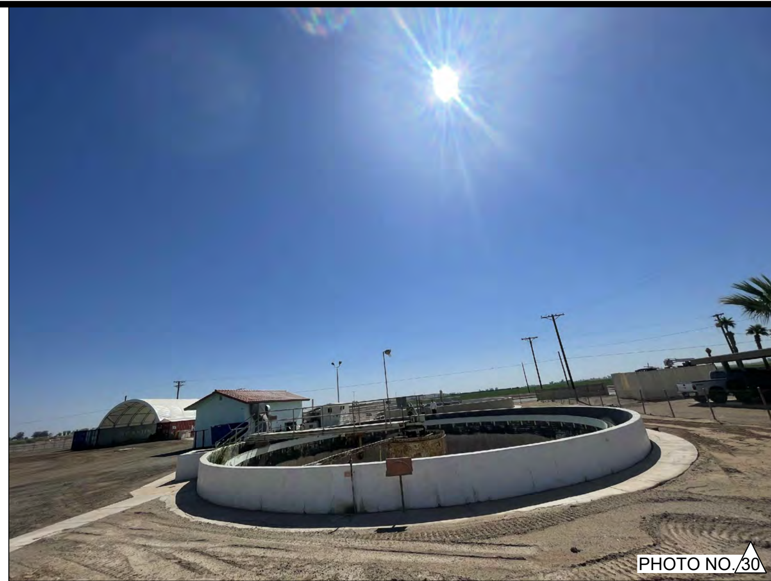
CLARIFIER NO. 1 - PHOTO OF THE WEST SIDE VIEW OF CLARIFIER NUMBER 1.
