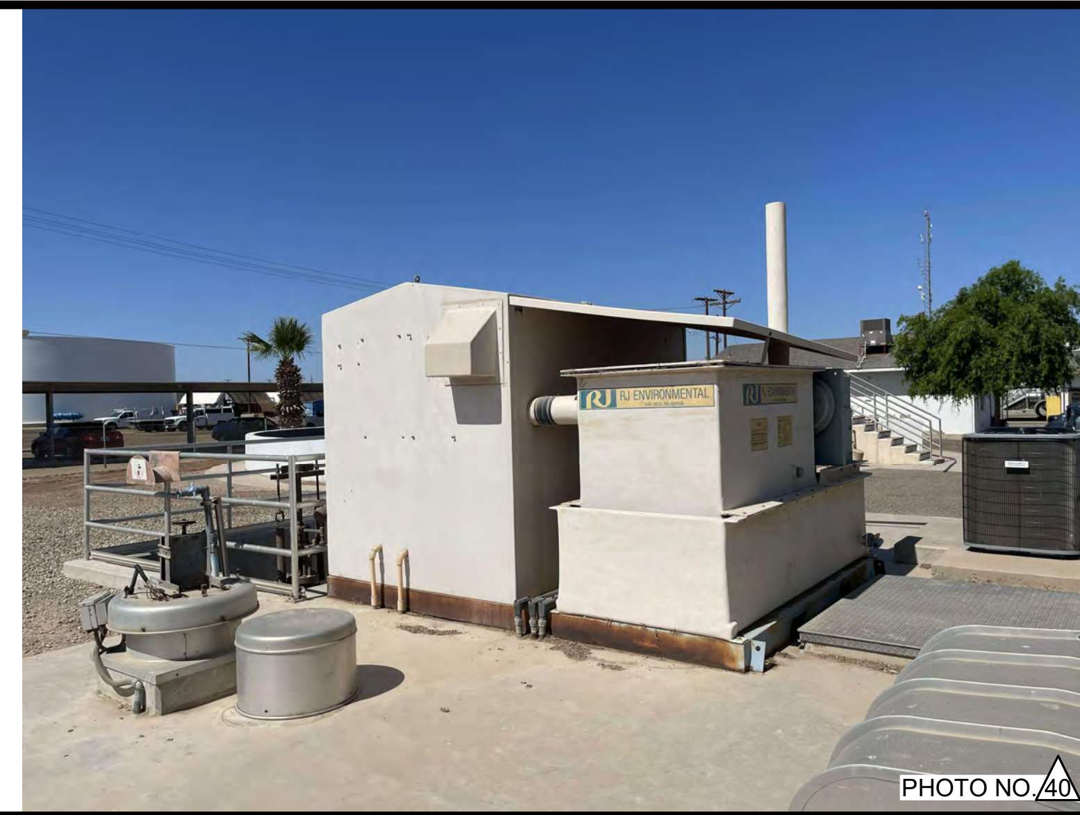
PHOTO OF THE MODULAR SCRUBBER AND CHLORINE FACILITY OF EXISTING SLUDGE PUMP STATION EXTERIOR GRADE LEVEL.
